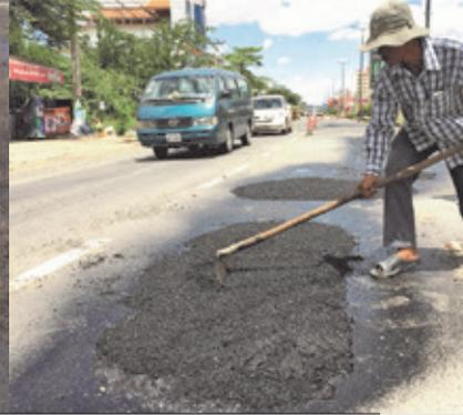
Packing Excel at IKEE's repair material-manufacturing facility in Cambodia (left). Road holes (middle) can be easily repaired using Excel cold mix asphalt (right).
