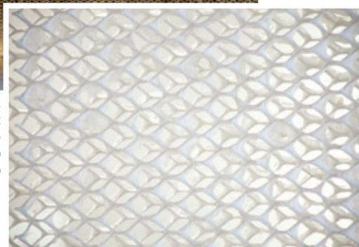
Japan, the cypress frame allows fresh air into the building while protecting the interior from direct sunlight. Reinforced by carbon fibers, the free-standing structure successfully creates the impression that an infinitely expanding forest has appeared in the heart of the city.
