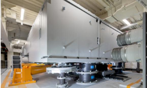
Close-up view of one of the TMD-NT vibration dampers: The Dual TMD-NT absorbs vibrations large and small. The double-staged rubber bearings support 700-ton steel weights.
