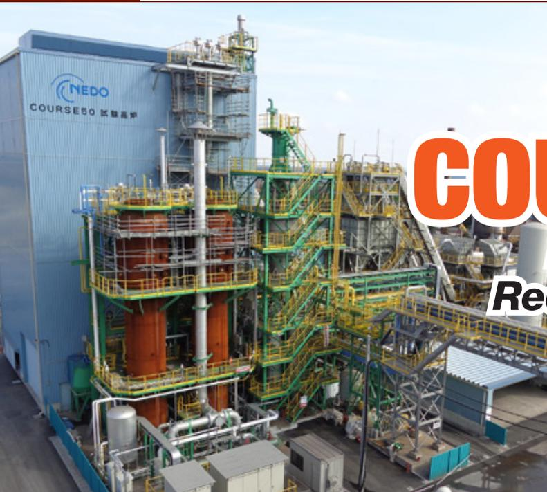
The experimental blast furnace equipment constructed at Kimitsu Works in Chiba Prefecture as part of the COURSE50 project. The blast furnace is installed inside the blue-colored building, which is approximately 30 m tall. Photo: Courtesy of NEDO
