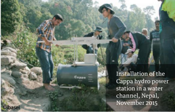
Installation of the Cappa hydro power station in a water channel, Nepal, November 2015
