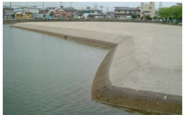
A levee constructed using soil improved using the Bon Terrain method
