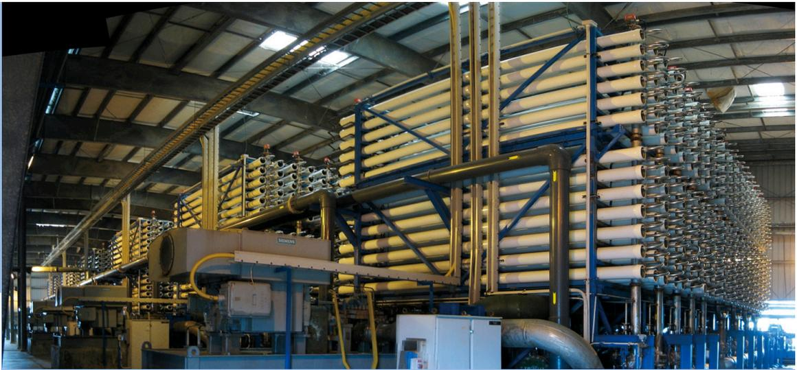
Mega-ton Water System reverse osmosis membrane module
