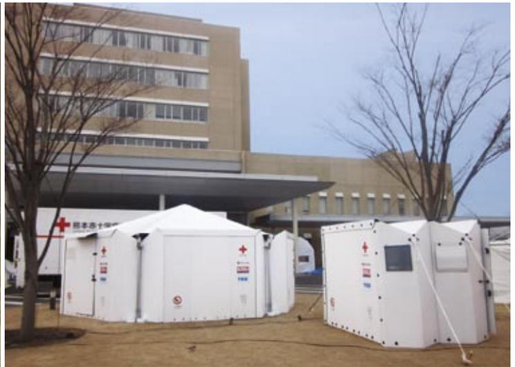
Temporary clinics set up with QS72 in front of a hospital in Ishinomaki, Miyagi Prefecture. The units are joined in a hexagonal pattern (right) and lengthways.
