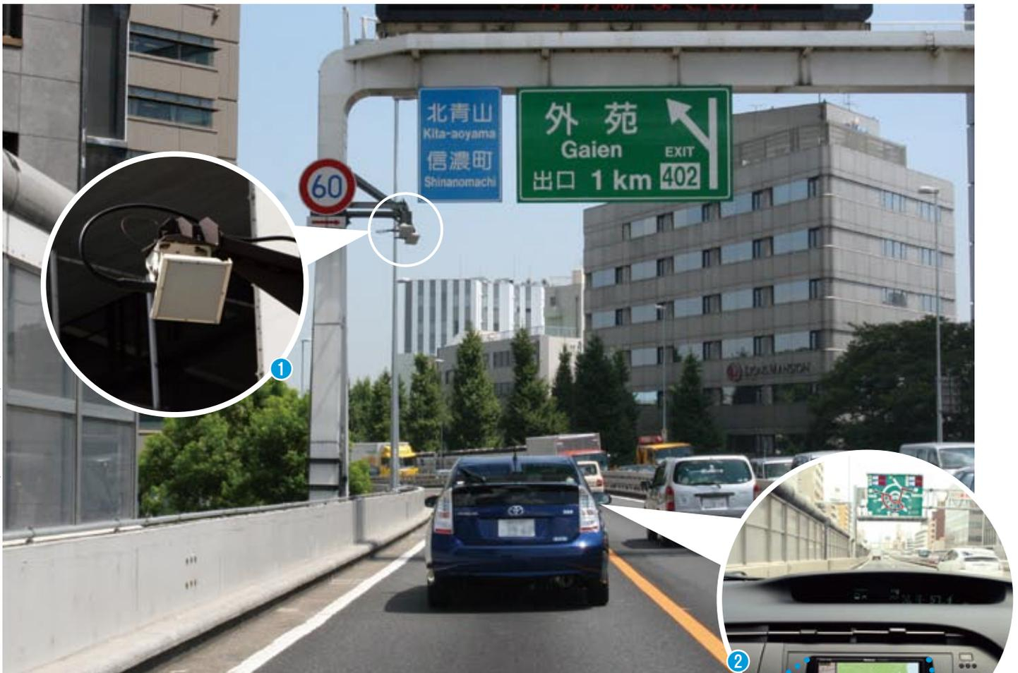
1,600 ITS Spot Units (1) have been installed on Japanese expressways. ITS Spot Service-equipped car navigation systems (2) automatically receive information such as the presence of obstacles on the road or congestion (3) and communicate it to the driver using real-time images (4).
